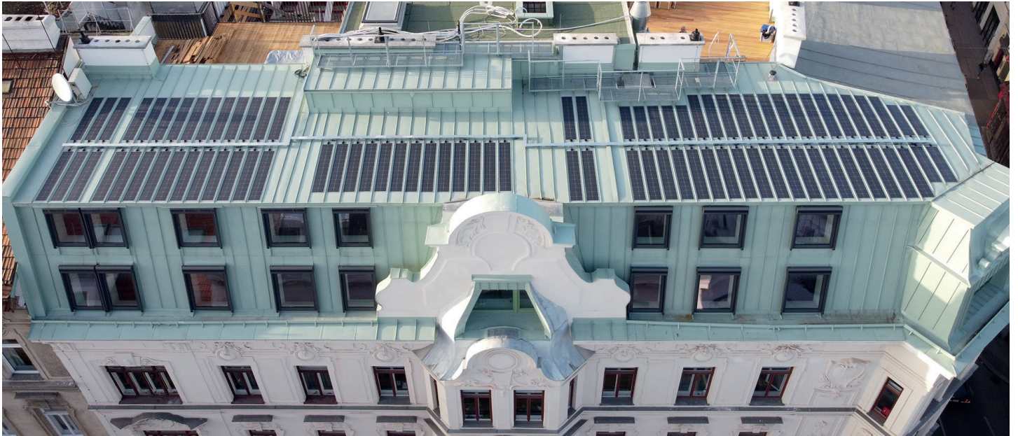
Rooftop installation private top floor
