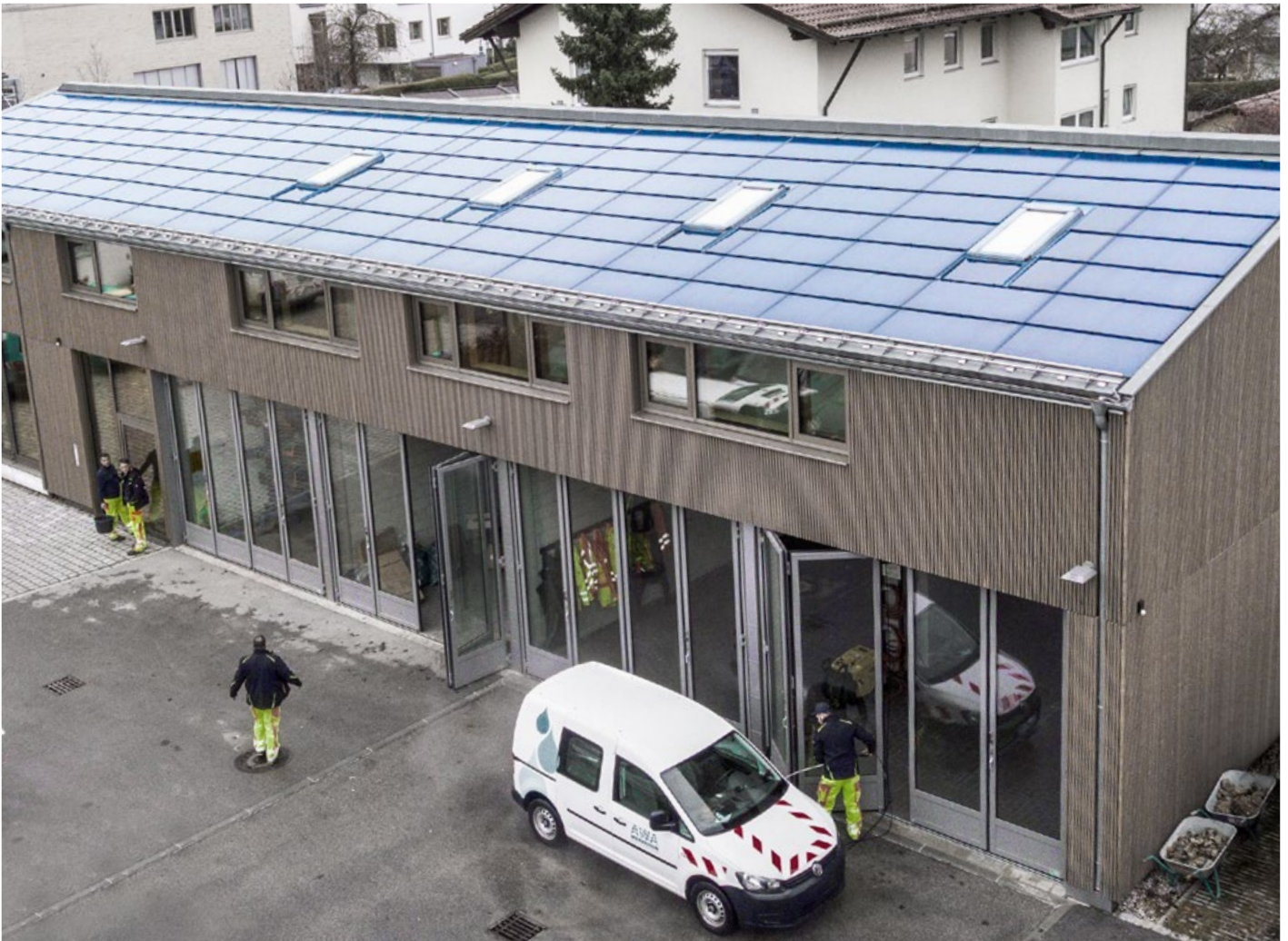
AWA-Ammersee Wasser- und Abwasserbetriebe gKU, operations building (municipal drinking water supply and wastewater treatment plant) Herrsching (Germany)
