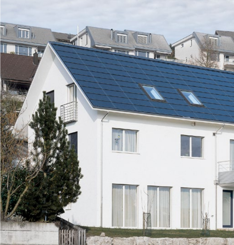
Single-family home Obersiggenthal (Switzerland)
